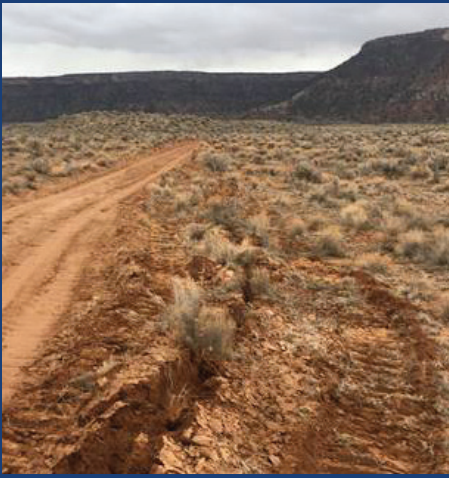
TRENCHING Scarring of environment
